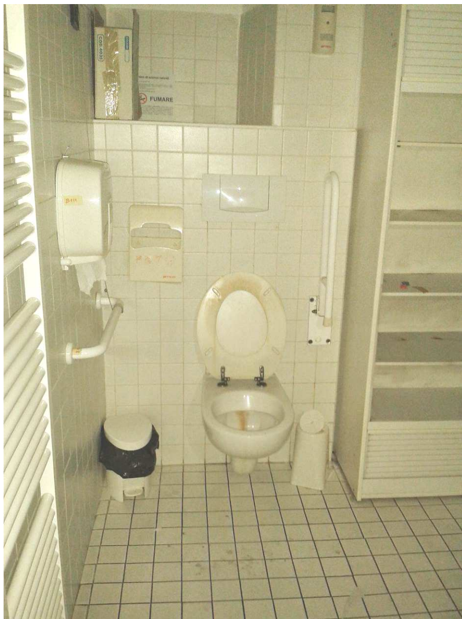
Piano Terra – bagno
